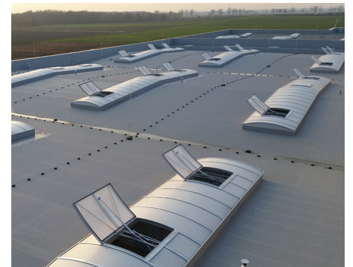
Fig. 4 - mcr PROLIGHT continous rooflights settled on warehouse
