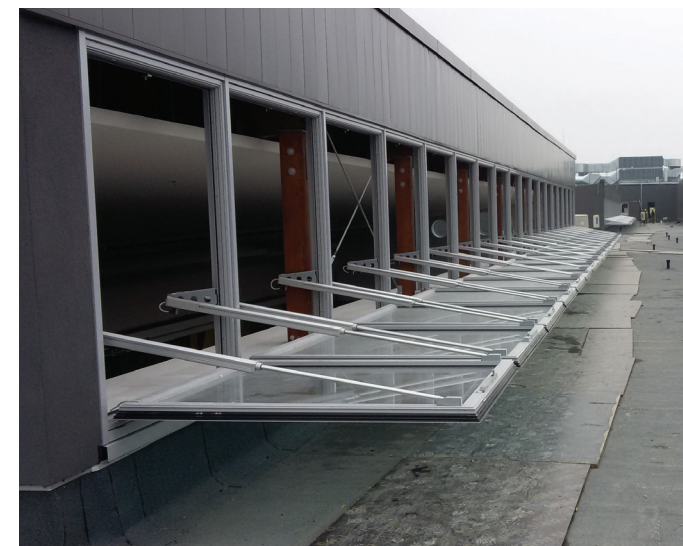
Fig. 34 - mcr OSO THERM smoke exhaust windows, open
