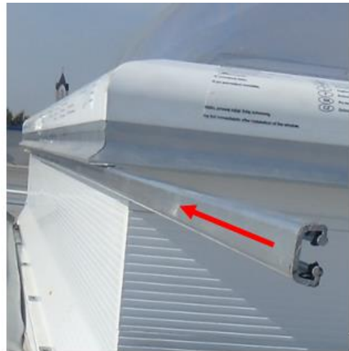
Fig. 18. Sliding the connector.
