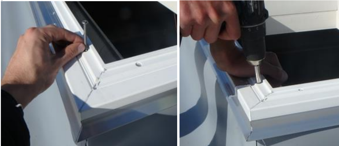
Fig. 10. Mounting of PVC frame to the metal base.
