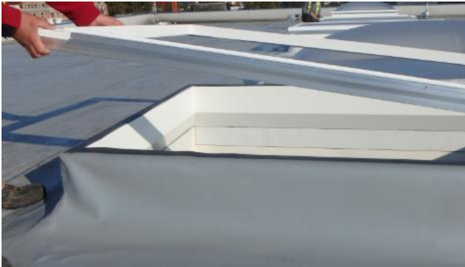
Fig. 9. Laying a PVC frame with a PES gasket.
