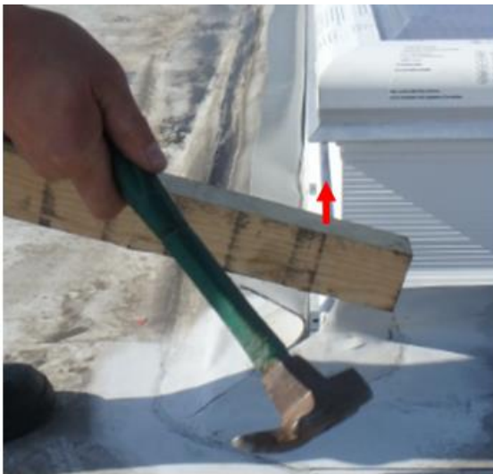
Fig. 19. Driving the connector.
