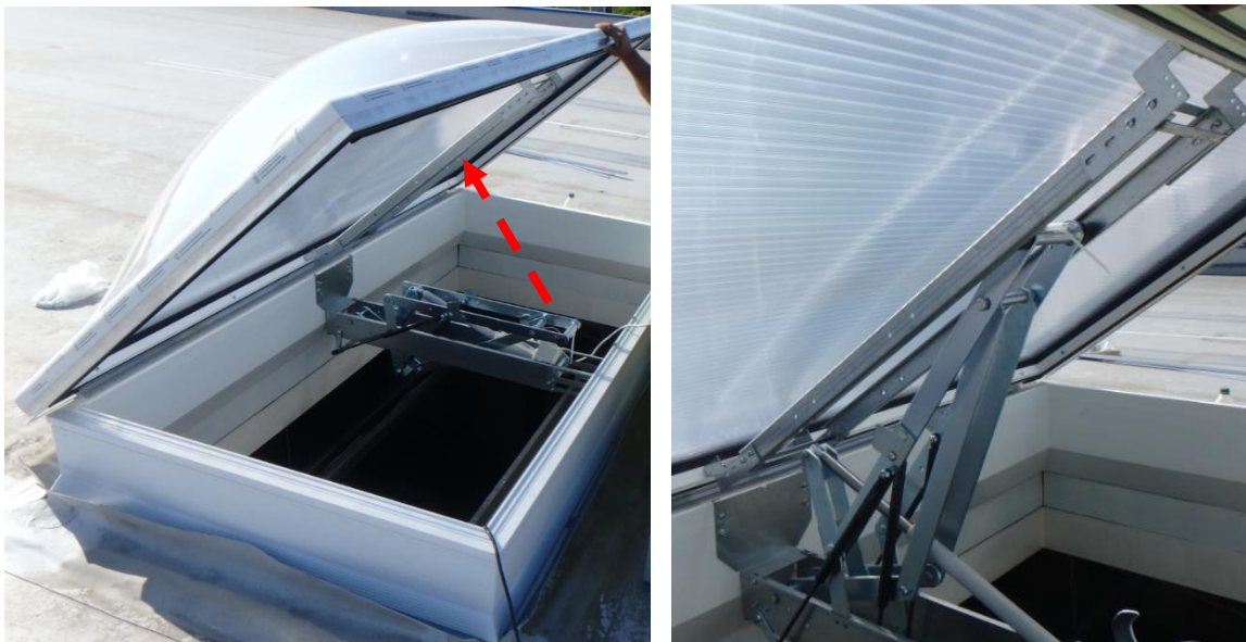
Fig. 28. Manually lift the vent leaf and open the mechanism to the crossbar height.
